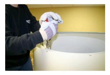
The tab locks the trim coil securely into the J-channel. Note that because the coil is not screwed into the support, this allows the aluminum to move slightly, helping with expansion and contraction issues. We punched each roll at about 6 - 8 inch intervals prior to installation (Figure 11).
