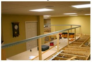
Since the backdrop was curved in so many places and the supports were rectangular, this caused a real problem when mounting the channel. Following the advice of a long -time model
