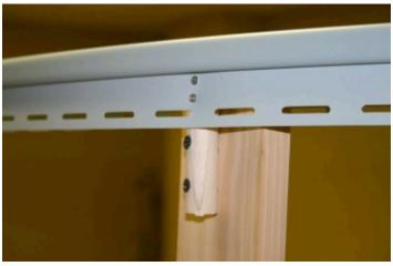
In curved areas where the rectangular nature of the upright would not allow the J-channel to be screwed securely, we also utilized dowels as spacers. See Figure 7.
